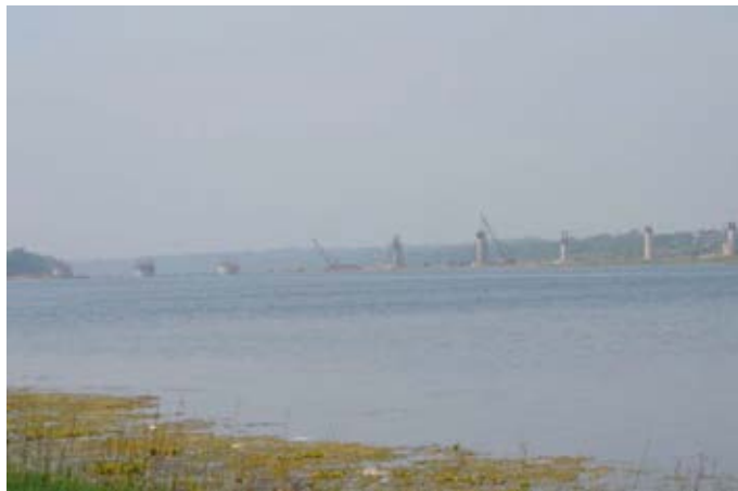
Figure 6. Bridge construction activity observed near sighting location
