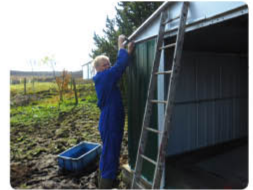
Paul working on the new shed
