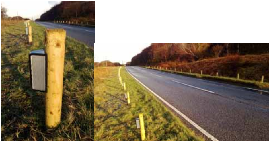
Figure 10. Reflectors at Pennygown: (a) showing reflector on post and 10(b) showing roadside positioning
